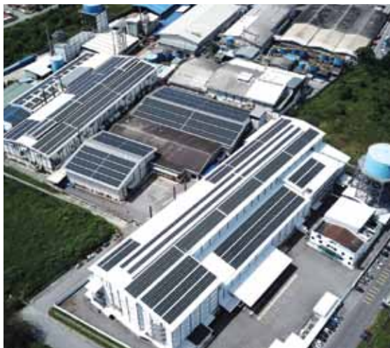
Solar panels installed at Hexcare's glove production plants in Ipoh, Malaysia
